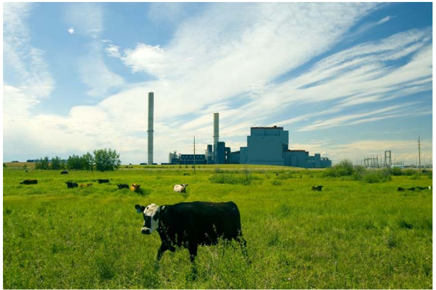
Genesee generating station
